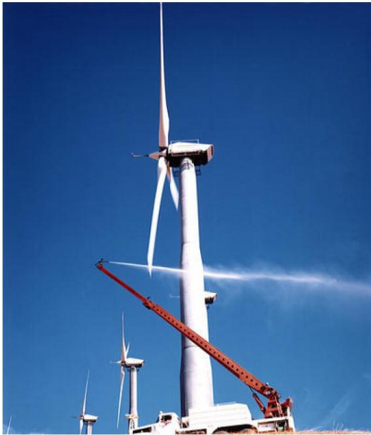
Washing a wind turbine at Altamont Pass, California
